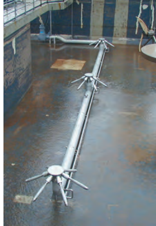
Aeration tank 1: ejectors DN200/6
