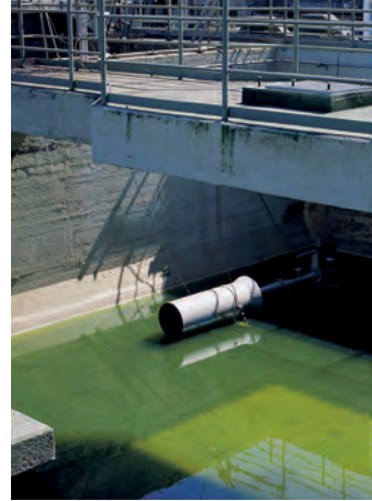
Aeration tank 3: SOLVOX® SI10
