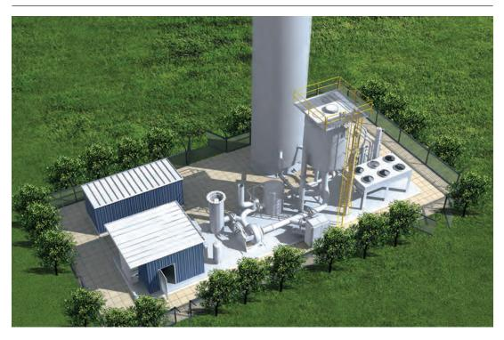
Linde's Vacuum Pressure Swing Adsorption (VPSA) oxygen systems are used in a variety of industries – metals, glass, cement, pulp & paper, refining, wastewater and mining. They provide lower unit cost and high reliability for customers requiring oxygen purity from 85-94%.
