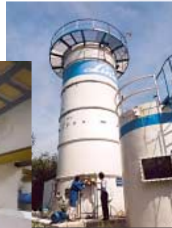
Water tower for testing and optimizing gas injection systems
