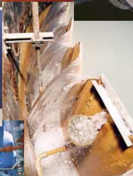
Overflow with lance for carbon dioxide injection
