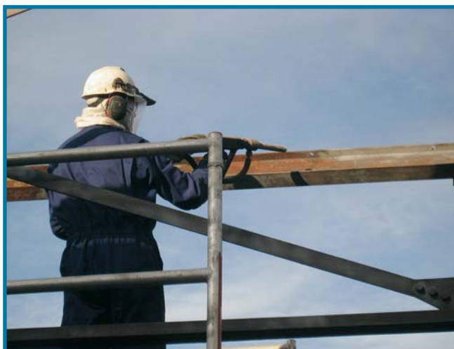
Fig. 4. "CryoAdd" proves during de-rusting of steel profiles.
